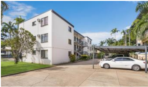
Unit 6, 8 Malabar Ct, Larrakeyah
