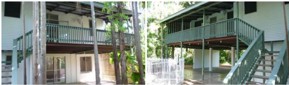
78 Nightcliff Road, Rapid Creek
